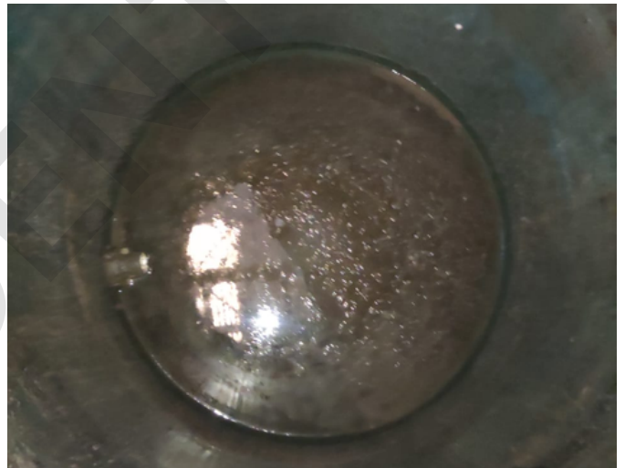
Sludge formation in the dosing tank
